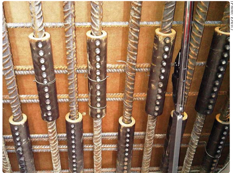
Above: 32mm MBT couplers in place. Below: Complex testing of coupled joint.
