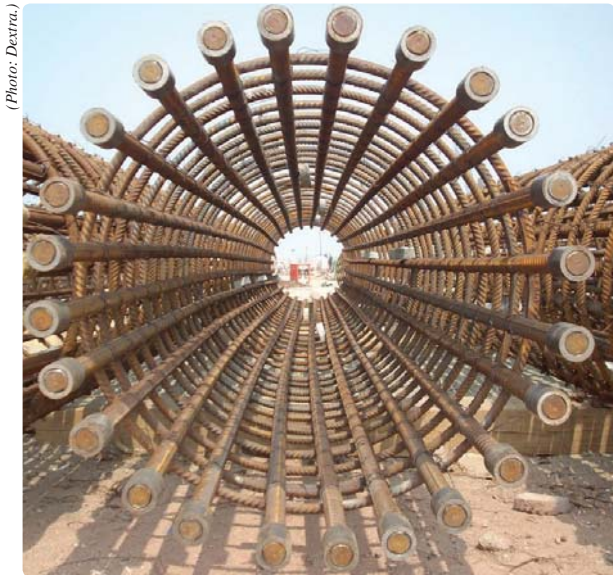
Couplers on a cage for a bored pile.
